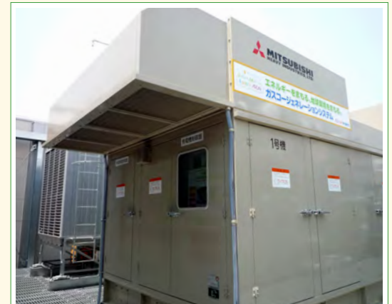
The gas cogeneration system for use during normal times as well as during emergencies uses medium-pressure gas, which is highly resistant to earthquakes, and becomes a source of power during electricity outages.
